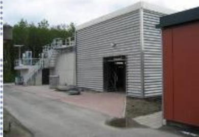
Netherland (Sewage, 2,400 m³/d)
